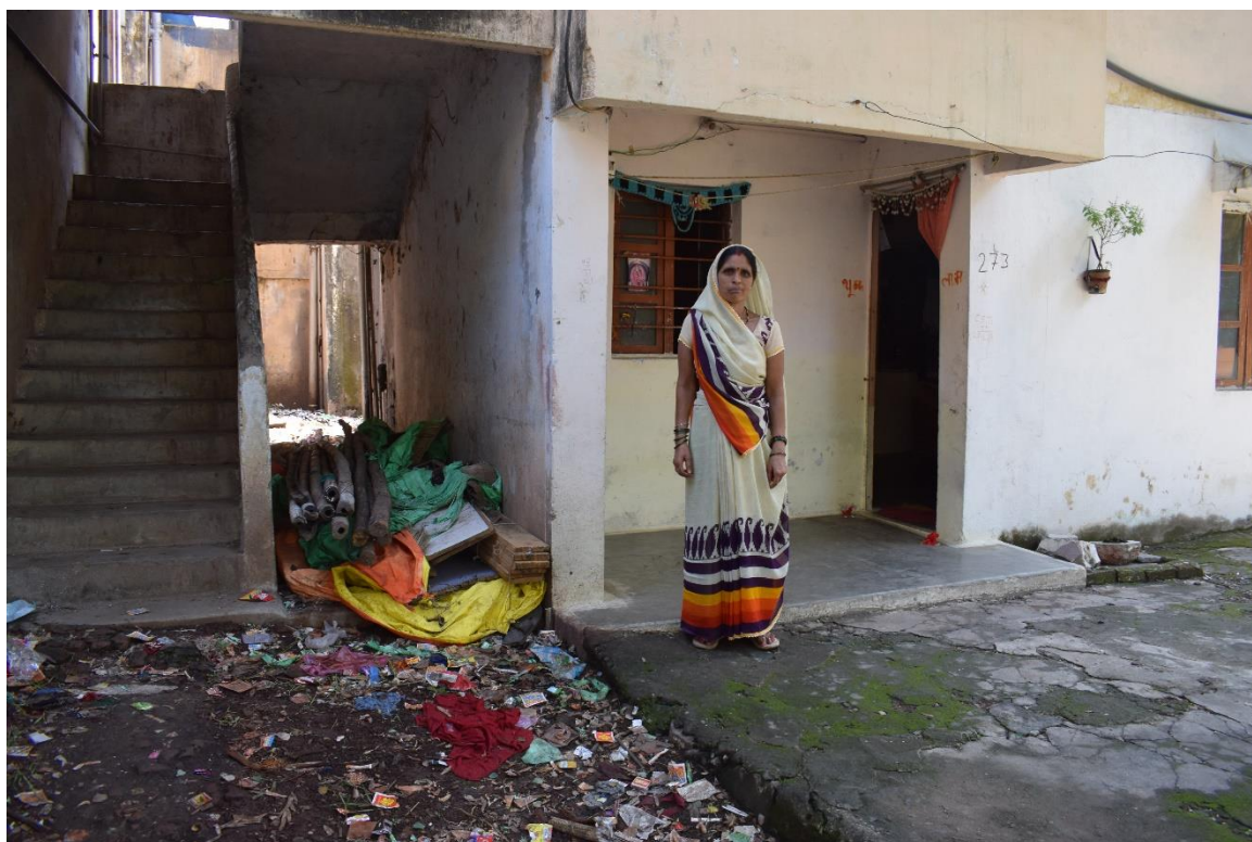
Fig 3.5. Waste dumped outside the Gas Widow Quarters
