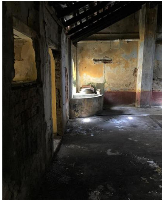
Figure 4: A bathroom inside Sassoon Hall, a 250-year-old house
