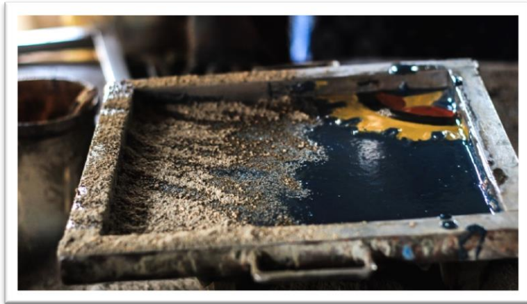
Fig 11: Adding the cement and Athangudi soil (Discover India Program, 2016)
